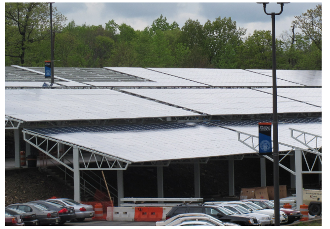
PHOTO SOURCE - © 2010 BIRDSALL SERVICES GROUP
