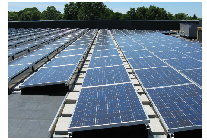
PHOTO SOURCE - © 2010 BIRDSALL SERVICES GROUP
