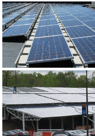
PHOTO SOURCE - © 2010 BIRDSALL SERVICES GROUP
