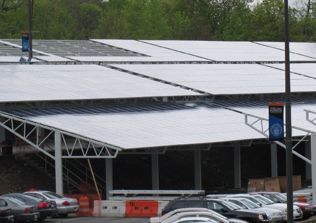
PHOTO SOURCE - © 2010 BIRDSALL SERVICES GROUP
