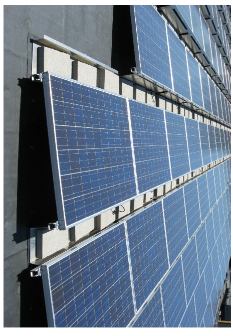
PHOTO SOURCE - © 2010 BIRDSALL SERVICES GROUP
