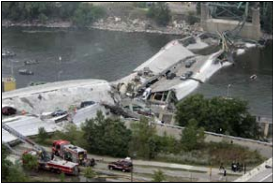
Minnesota Bridge Failure
