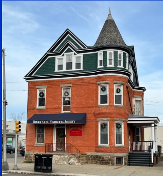
Arthur W. Condict House Exterior Restoration Location: Town of Dover Grant: $144,576
