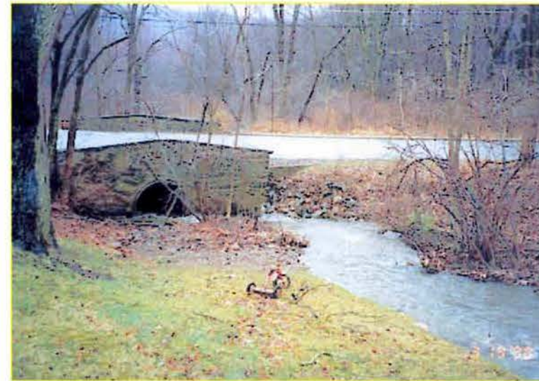
VIEW OF EXISTING UPSTREAM FACE OF ST. MARY'S AVE. 48" \phi RCP CULVERT
