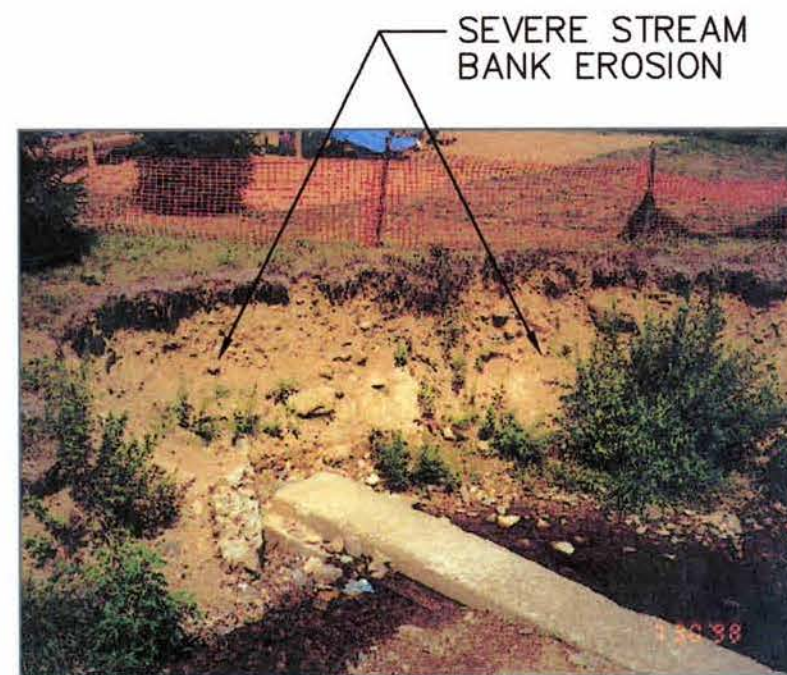
VIEW OF EXISTING SCOUR HOLE TO BE REPAIRED WITH LARGE BOULDERS
