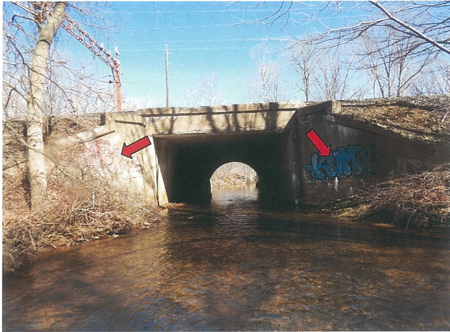
PHOTO 5-1: South elevation, looking north. Note tree growth in front of the southwest wingwall and graffiti (arrows) at the southeast and southwest wingwalls.
