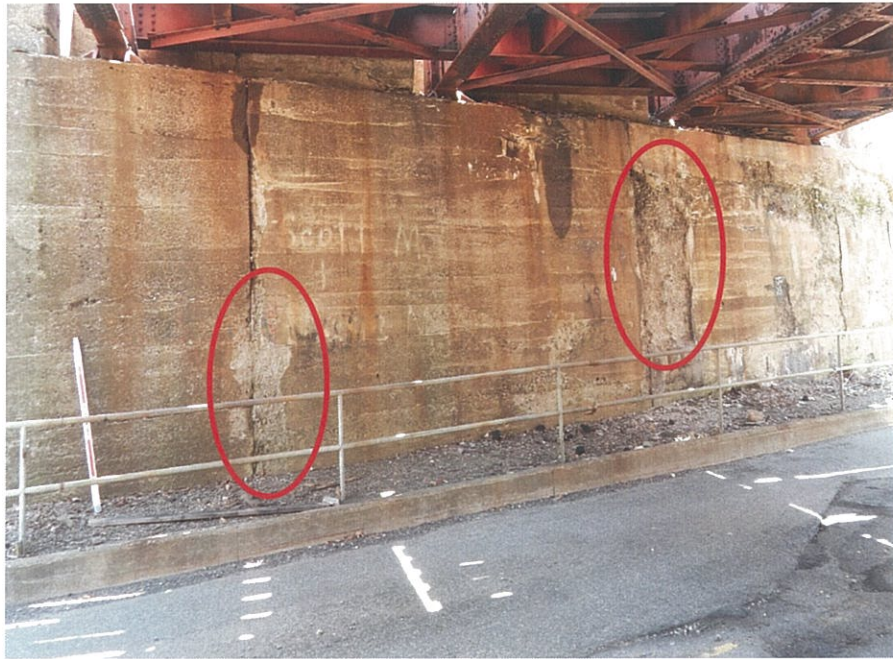
PHOTO 5-7: General view of the east abutment, looking east. Note the large spalls and delaminated concrete throughout the abutment (Circles).
