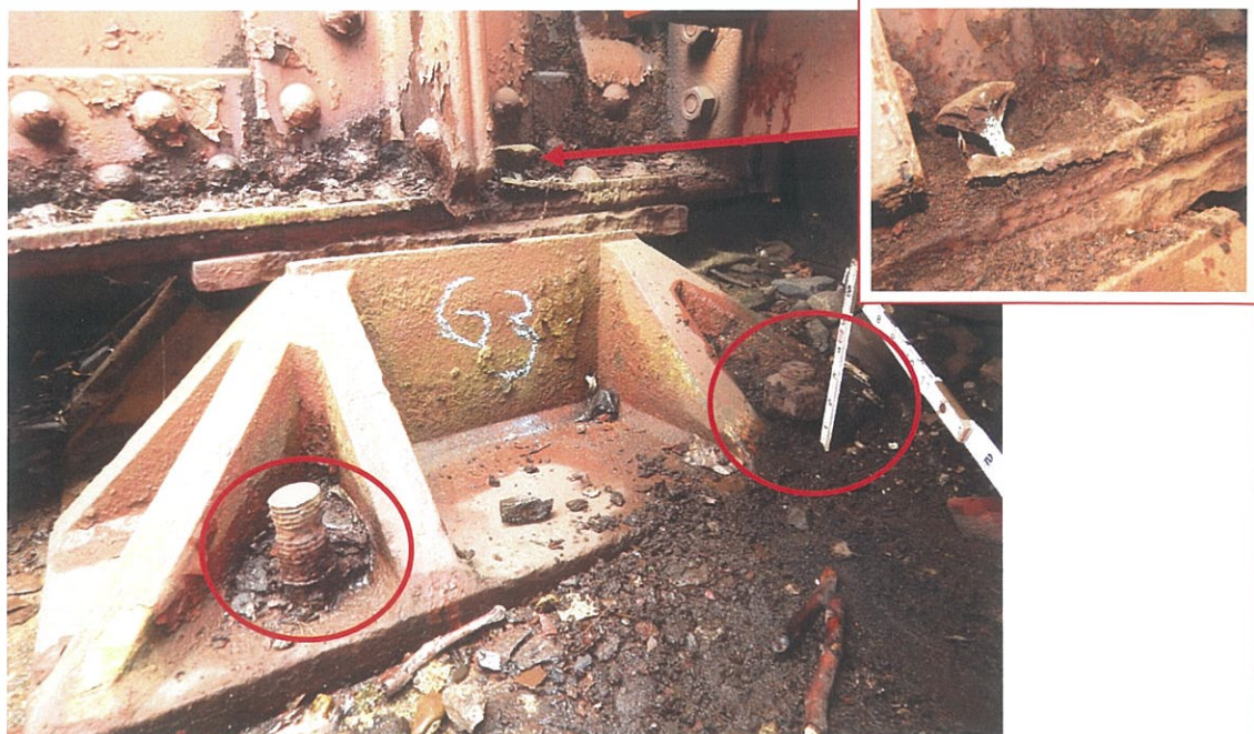
PHOTO 5-16: Missing and raised anchor bolt nuts (Circles) at the north side of Girder G3 bearing over the west abutment, looking southwest. Note up to 100% section loss to the sole plate bolt (Insert). Note also, the bearing is seized.
