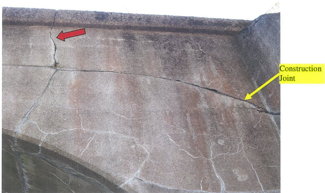
PHOTO 5-10: Wide crack at west end of the north spandrel wall, looking south (arrow). Note fine map cracks with efflorescence.
