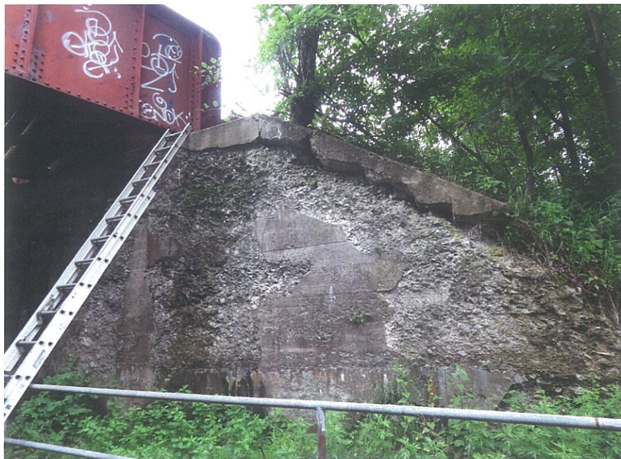
PHOTO 5-18: Large spalls and delaminated concrete throughout the southeast wingwall, looking northeast. Note tree growth behind the wingwall.
