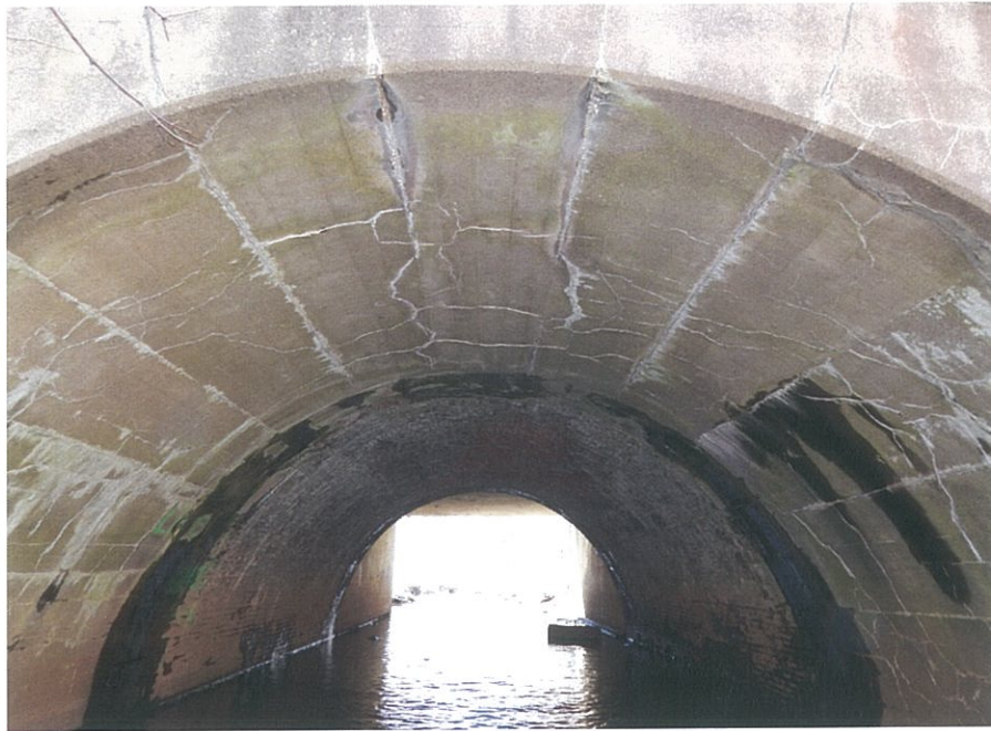
PHOTO 5-7: General view of intrados of concrete and brick arches, looking south. Note several fine cracks with efflorescence, water staining and active water leakage at the concrete arch intrados. Note also, heavy efflorescence throughout the brick arch.
