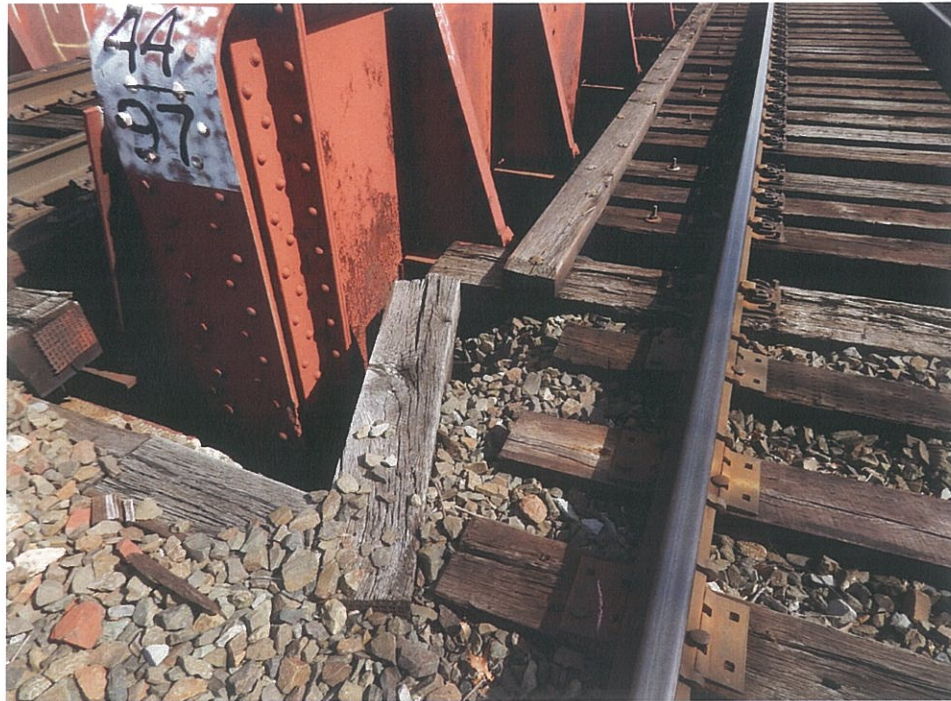
PHOTO 5-13: Displaced ballast retainer at the west end of Girder G3 on Track #2, looking northeast.
