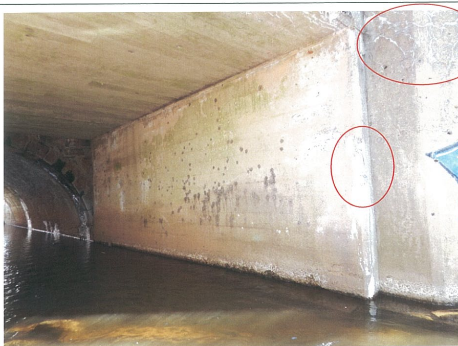
PHOTO 5-8: General view of the east abutment breastwall of concrete slab, looking northeast. Note fine cracks with efflorescence at top of the southeast wingwall. Note also, small spall with heavy efflorescence along the south edge, approximately located at mid height of the breastwall.
