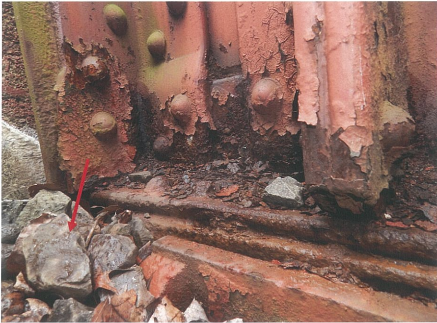
PHOTO 5-17: Missing sole plate bolt at the north side of Girder G3 bearing over the east abutment, looking southeast. Note the accumulation of ballast on the bearing seat.
