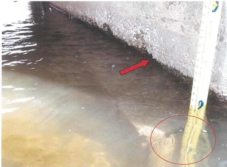
PHOTO 5-11: Moderate to severe scaling along the bottom of east abutment breastwall of concrete deck slab, looking northeast. Note exposed footing at south end (typical throughout the length of the breastwall).
