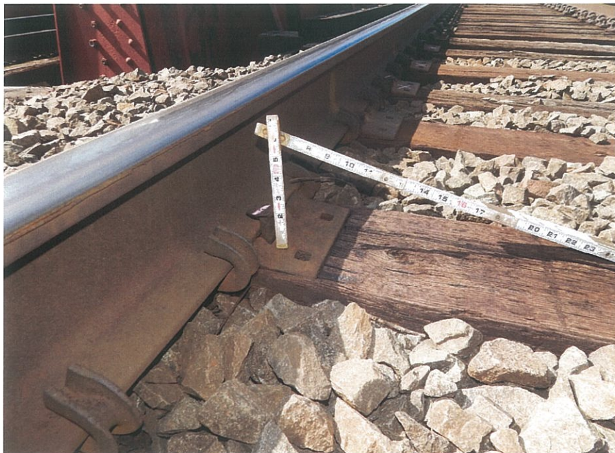
PHOTO 5-12: Raised spike at the south rail on Track #1 at the east approach, looking southwest.
