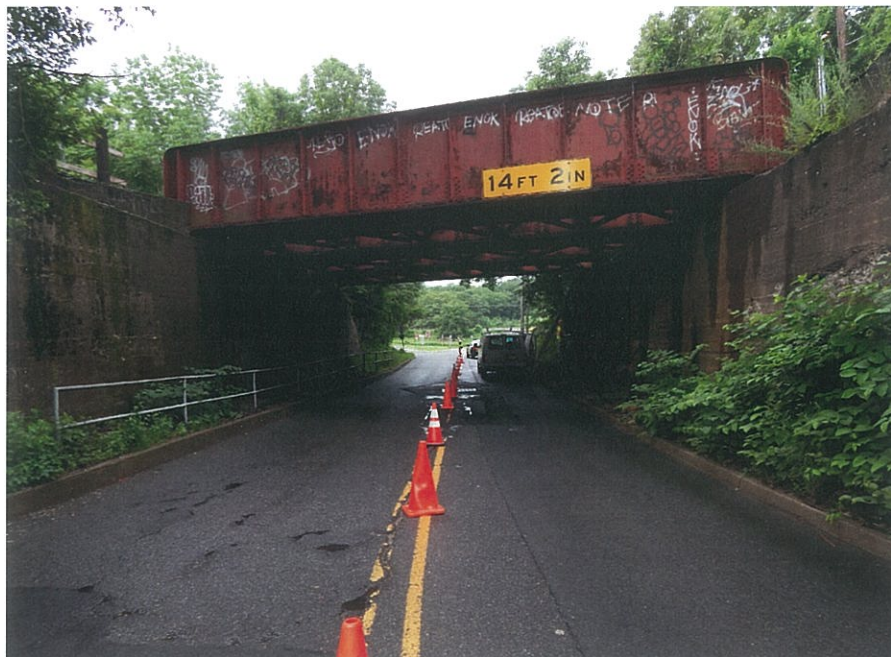
PHOTO 5-2: North elevation, looking south. Work Done: 14'-2" Vertical clearance sign has been installed at the north fascia.
