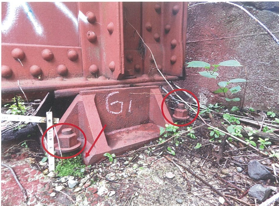
PHOTO 5-8: General view of bearing G1 over the east abutment, looking northeast. Note raised anchor bolt nuts (Circles) and broken masonry plate at the southwest corner of the bearing (Arrow).
