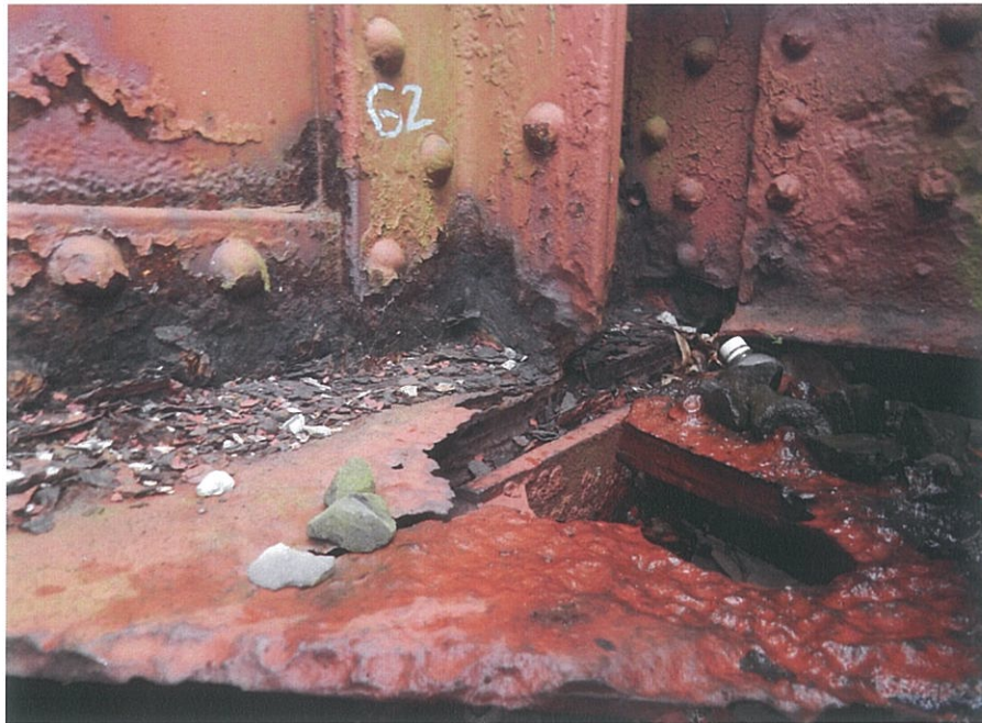
PHOTO 5-15: Severe section loss and holed through gusset plate at the south side of Girder G2 bearing over the east abutment, looking northeast.
