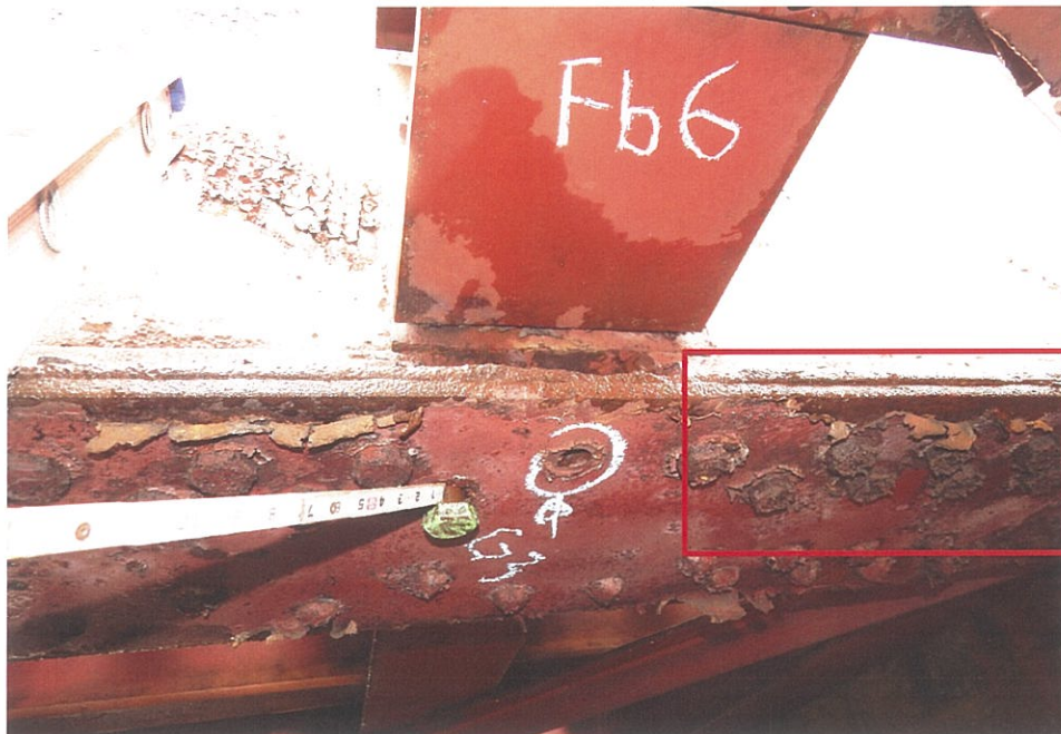
PHOTO 5-14: Missing bolt and loose bolt at the bottom flange of Girder G3 at Floorbeam FB6, looking south. Note the rivets at the bottom flange of Girder G3 exhibit greater than 50% head loss (Rectangle).
