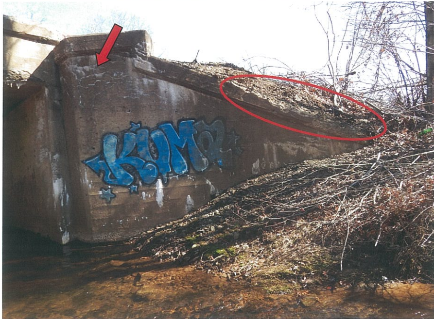
PHOTO 5-13: Large spall (circle) along the top face of the southeast wingwall, looking northeast. Note scattered fine cracks with efflorescence (arrow) at the vertical face of the wingwall.
