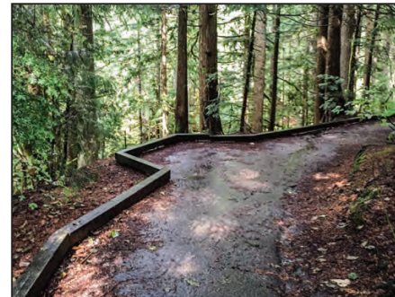
Trail Class 5: Tread —The tread is wide, firm, stable, and generally uniform. Trails are commonly hardened with asphalt or other imported material.
