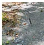
Figure 1: Erosion of loose aggregate trail.
