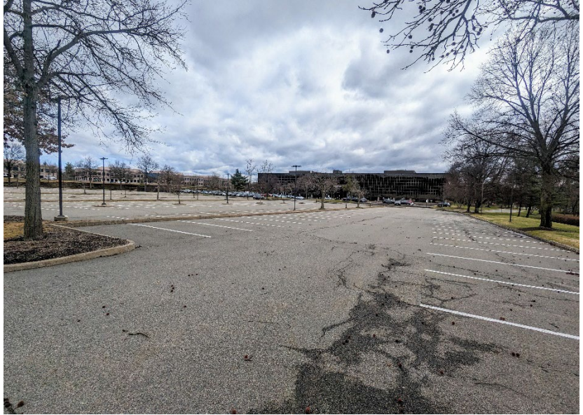
FIGURE 1: PARKING LOT AT 4 CAMPUS DRIVE (3/7/2024).
