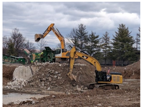
FIGURE 3: DEMOLITION OF 2 CAMPUS DRIVE (1/26/2023)
